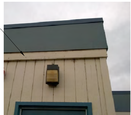
P14 EAST FLASHING
